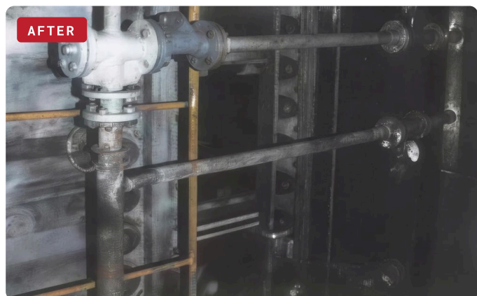
After the retrofit: a higher, more even surface temperature.
